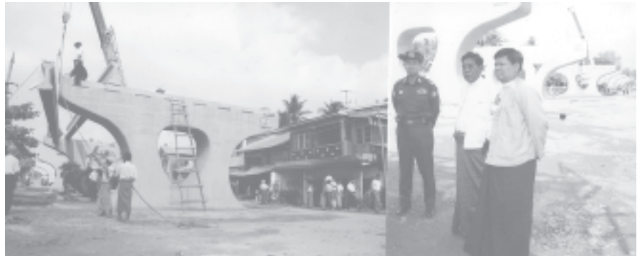
Rail Transportation Minister Maj-Gen Aung Min inspects progress of Kyaukyedwin overpass.—MNA
