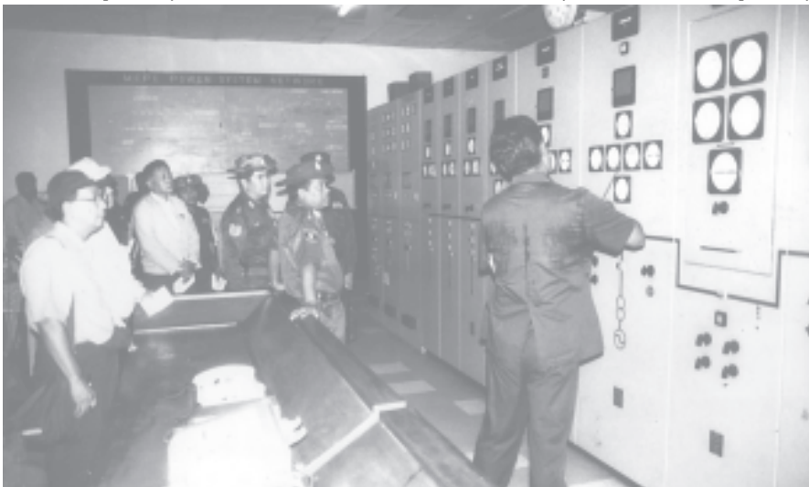
Lt-Gen Ye Myint inspects power control room at power plant.—MNA
