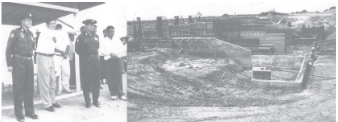
Lt-Gen Khin Maung Than inspects construction of Moeyungyi Sluice Gate in Waw Township — MNA
