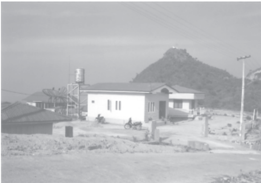
Communication Station of Thandaung Hill Station.
