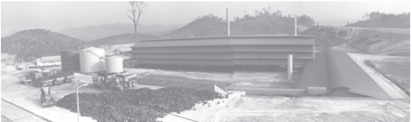
View of Crude Palm Oil Mill in Khamaukkyi, Kawthoung Township.— MNA
