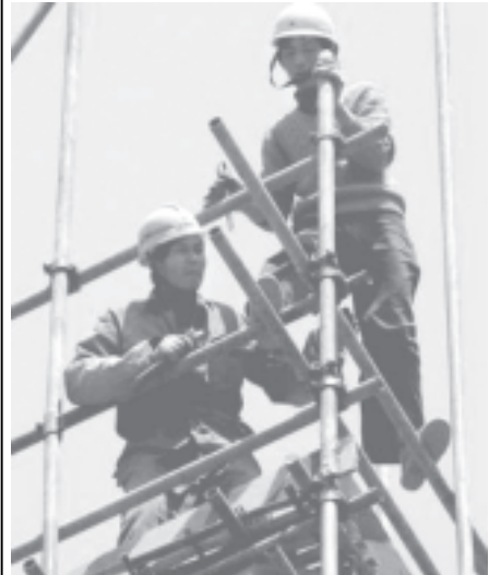
Chinese construction workers install metal scaffolding at a new property building being erected in Shanghai's business district on 4 April, 2005.—INTERNET
