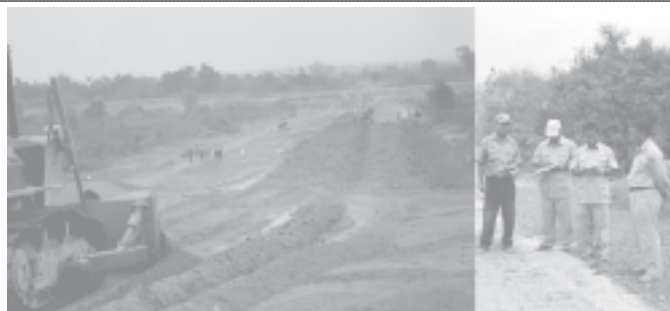
Director-General U Myo Myint inspects district-to-district road in Taikkyi Township. — MNA
