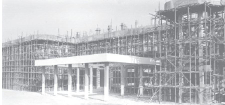
Convocation Hall of Mawlamyine University under construction. — MNA
