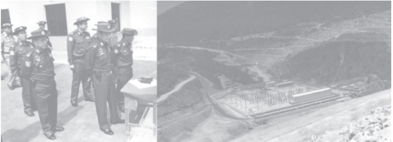
Vice-Senior General Maung Aye views the underground power plant from Paunglaung Multi-purpose Dam. — MNA
