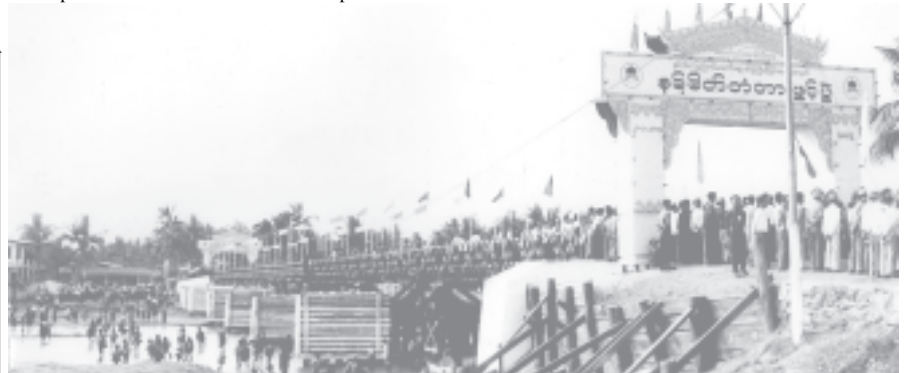
With the length of 376 feet, Namtmeik Bridge in Momeik, Kyaukme District, is a bailey type.—MNA
