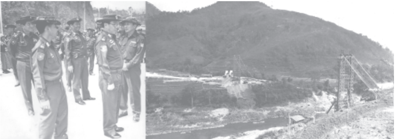
Prime Minister Lt-Gen Soe Win inspects installation of Thanlwin Suspension Bridge (Tarpa). —MNA
