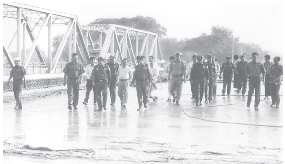
Lt-Gen Ye Myint views round the construction site of Myitnge River Bridge (Mandalay).— MNA
