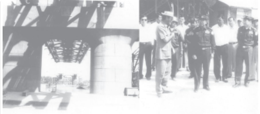
Minister for Construction Maj-Gen Saw Tun inspects construction of Pyapon Bridge.— CONSTRUCTION
