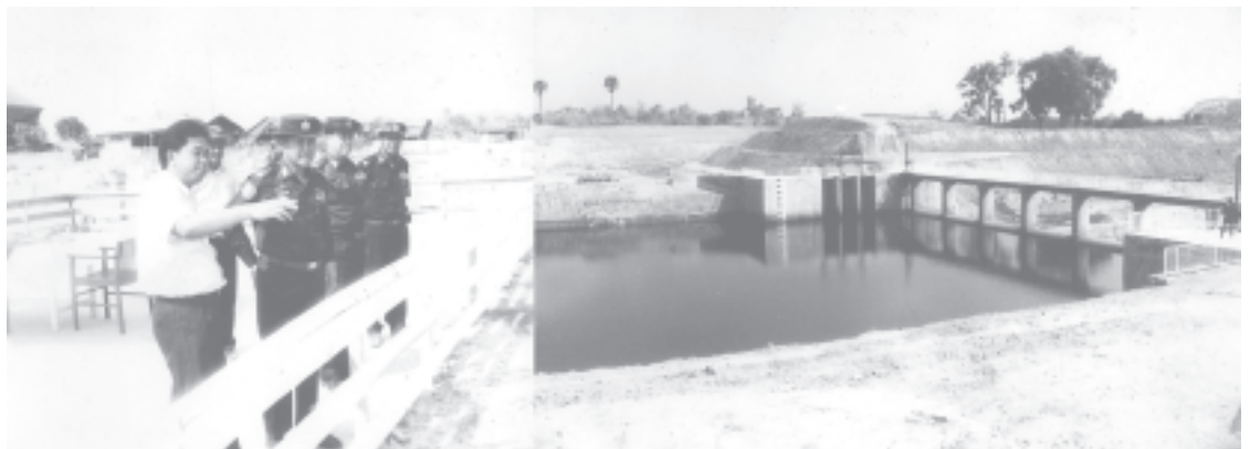
Lt-Gen Khin Maung Than inspects progress of building Thonze Dam Project in Thayawady Township.—MNA
