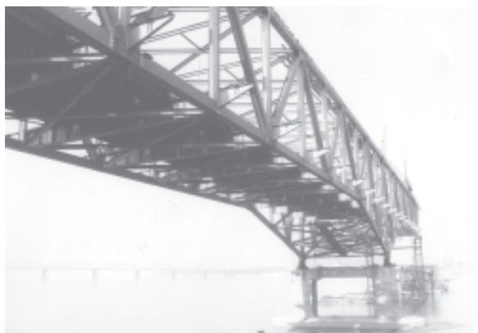
Progress of installation of iron beams in Ayeyawady Bridge (Yadanabon). — MNA
