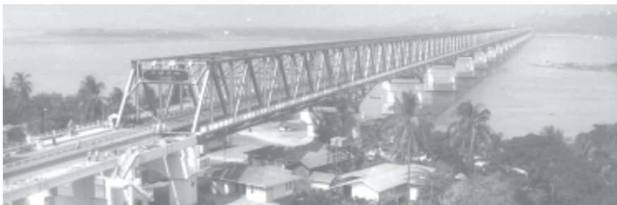
The 11,575-foot rail-cum-road Thanlwin Bridge (Mawlamyine), the longest and the largest in Myanmar, lies on Thanlwin River after its opening ceremony. — MNA
