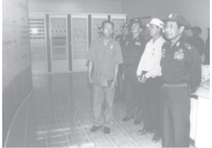
Vice-Senior General Maung Aye inspects power control room of Thaphanseik Hydel Power Plant.—MNA
