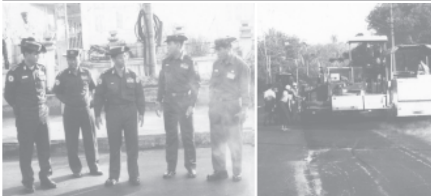
Commander Maj-Gen Myint Swe views the tarmacking of the road in front of Olympic Tower on Strand Road, Ahlon Township. — YGN COMMAND
