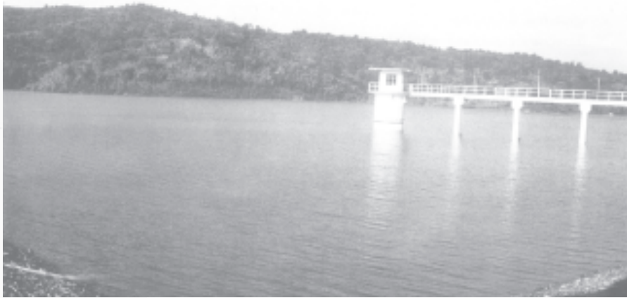
Nankathu Dam in Ingapu Township, Ayeyawady Division. — MYANMA ALIN
