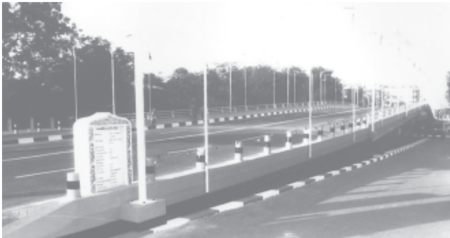
The newly-opened Nanattaw Overpass in Kamayut Township.— MNA
