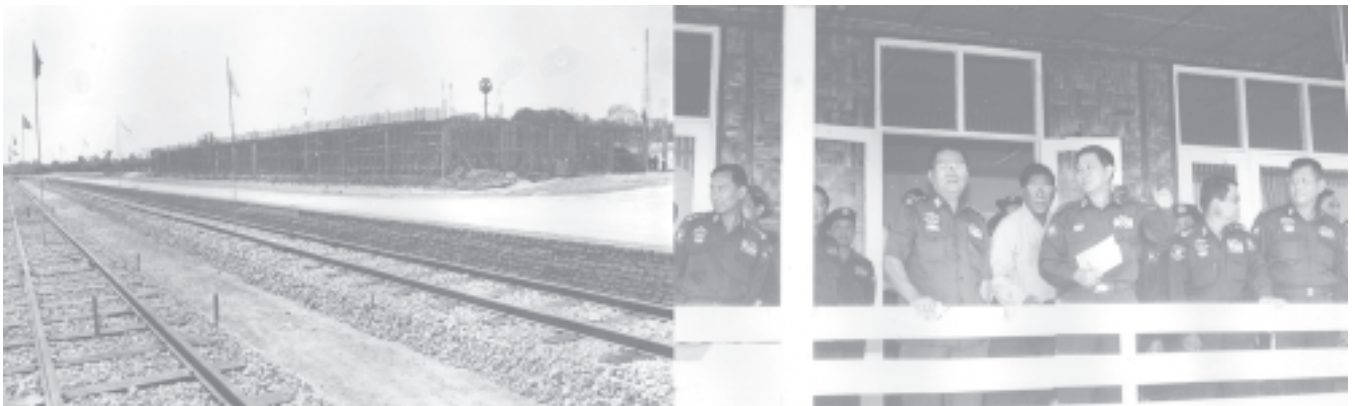
Senior General Than Shwe inspects progress in construction of Mawlamyine Railway Station and laying rails. — MNA
