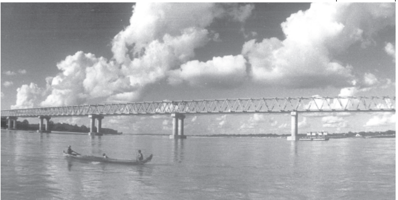
With the length of 4320 feet, Chindwin Bridge (Monywa) spans Chindwin river in Monywa Township, Sagaing Division. MYANMA ALIN
