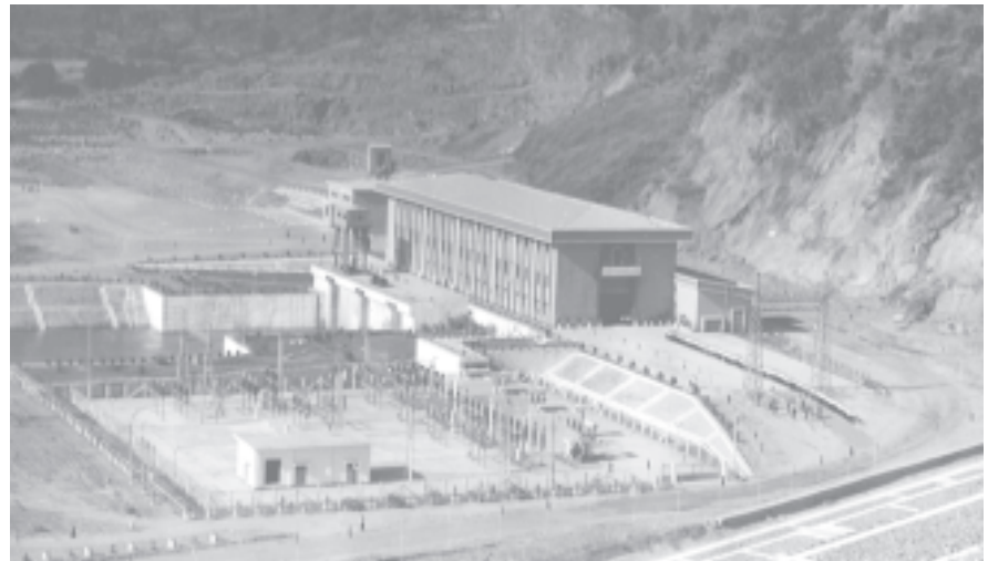
The Mone Creek Hydel-power Plant. — MNA
