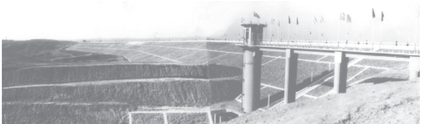
Pade Dam on the Pade Creek in Aunglan Township, Thayet District, Mangway Division.—MNA
