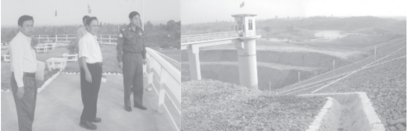
Minister Maj-Gen Htay Oo inspects the spillway of Pade Dam being constructed in Aunglan Township. — AGRI & IRR
