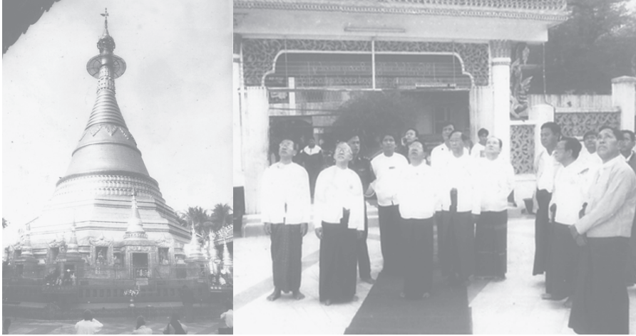
Minister Brig-Gen Kyaw Hsan inspects tasks for all-round renovation of the Shwephonepwint Pagoda. — MNA
