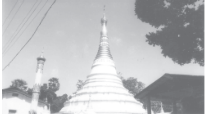
The Kyaikbodhi Pagoda seen after being renovated. — MNA
