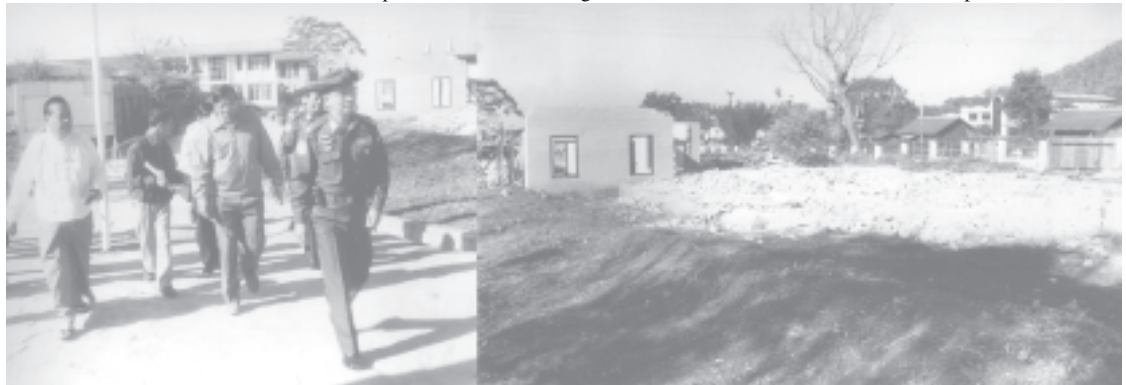
Secretary-1 Lt-Gen Thein Sein inspects the construction site of the three-storey annexe to Women's and Children's Specialist Hospital in Taunggyi.—MNA .
