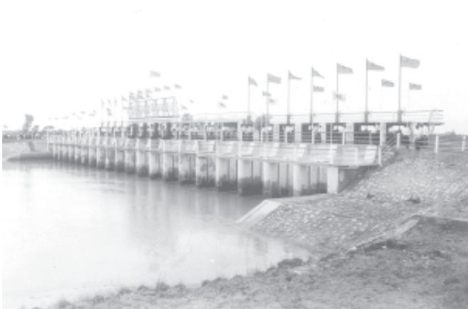
Zaikkaye Sluice Gate with 21 valves, each of which measures 6 feet by 12 feet, is of concrete type and was opened on 25 June 2002 near Zaikkaye canal in Aungkantha village, Thaton Township, Mon State. It can supply water to 20,000 acres of farmland in the region.
