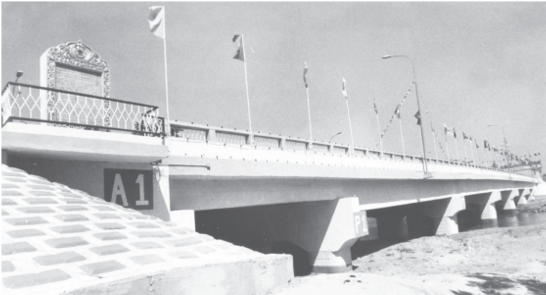
Daka Bridge which was opened on 6 July 2003 on Yangon-Pathayin road is 1400 feet long and has 28 feet wide motorway with 5 feet wide pedestrian lanes on both sides. — PHOTO: MNA
