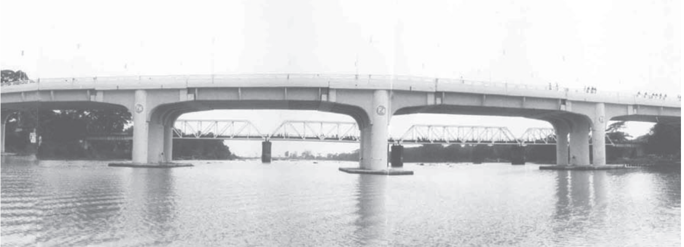
Daka Bridge which was opened on 6 July 2003 on Yangon-Pathayin road is 1400 feet long and has 28 feet wide motorway with 5 feet wide pedestrian lanes on both sides. — PHOTO: MNA
