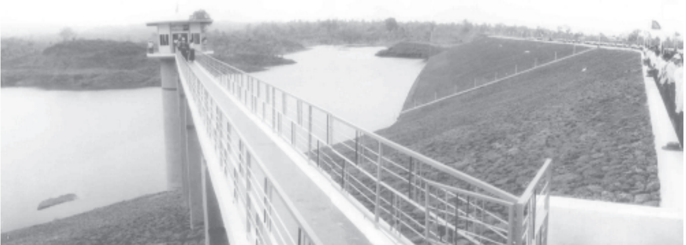
Water is essential not only for agricultural purpose but also for household use. The Ministry of Agriculture and Irrigation is taking responsibilities for building dams and reservoirs in the country. The 132 feet high and 3,044 feet long Minhla Dam in Okpo Township will irrigate 5260 acres of farmland in Okpo Township and 9740 acres of cropland in Minhla Township.— PHOTO: MNA
