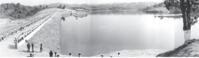
Hinywet Dam in An Township, Rakhine State. The dam was opened on 29-10-2002. With 750 feet in length and 70 feet in height, the dam was built at a cost of about K 100 million to supply water to about 100,000 people.
