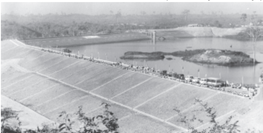
KALIHTAW DAM IN HLEGU TOWNSHIP, YANGON DIVISION: The Kalihtaw Dam was built at a cost of K 441 million. It can store 26,000 acre-ft of water and irrigate 9,000 acres of farmland. —MNA
