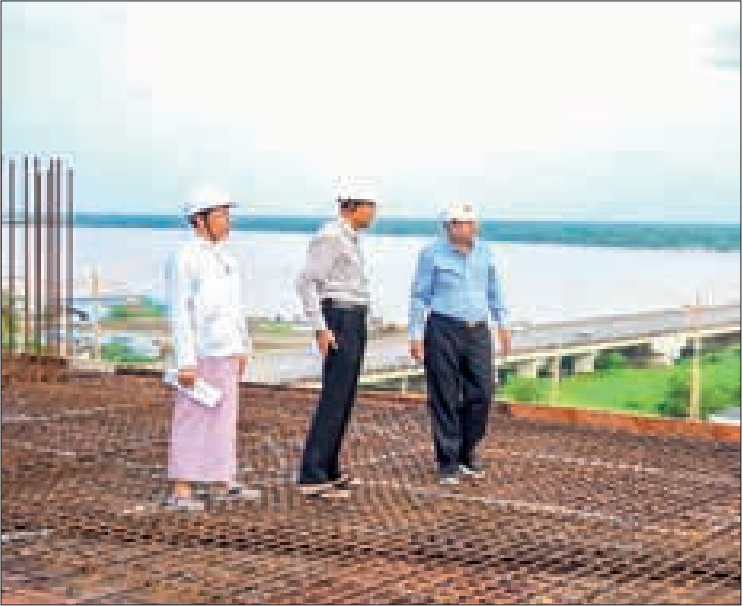
Deputy Minister U Myo Myint inspects the progress of the construction at the Oncology Unit of the National Cancer Treatment Centre in Yangon Region yesterday.
