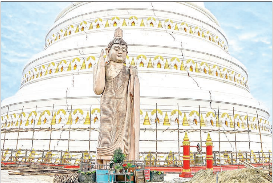
Bamboo scaffoldings are under preparation to repair the Htupayon Pagoda.
