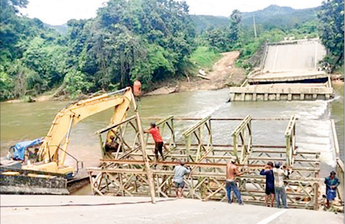
This image shows repair work on the Kawnwe Bridge along the Myawady-Kawkaik Asia Highway, disrupted by a terrorist suicide drone attack.
