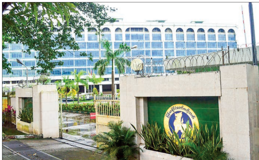
The general view of the Central Bank of Myanmar (CBM) office in Yangon.
