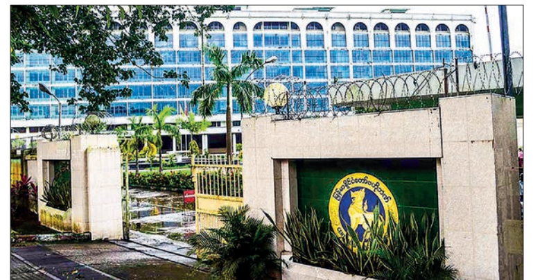
The general view of the Central Bank of Myanmar (CBM) office in Yangon.
