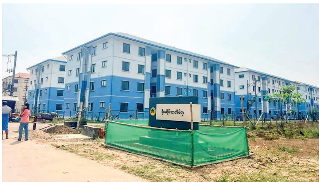
A general view of the Yoma low-cost housing and flat units.
