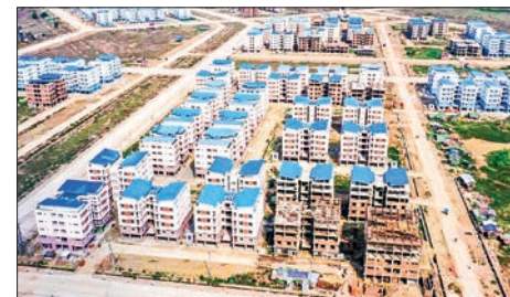
This photo captures apartments at the Thukha Dagon Housing.
