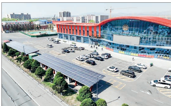
File photo shows electric vehicle (EV) charging piles in a highway service area in Taiyuan, north China's Shanxi Province.
