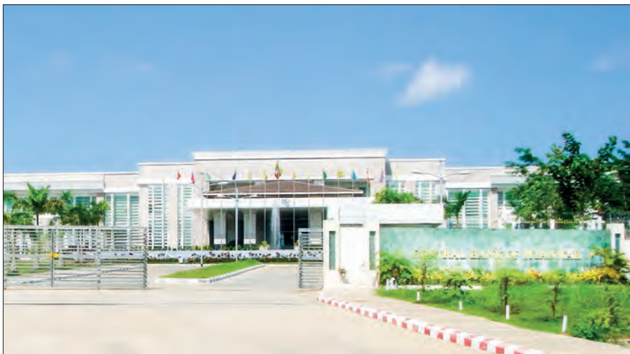
The general view of the office of the Central Bank of Myanmar in Nay Pyi Taw.
