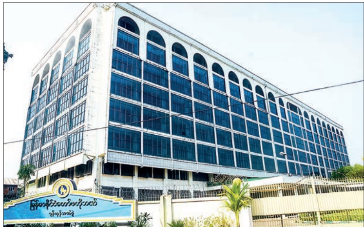
The facade of the Central Bank of Myanmar (Yangon Branch).
