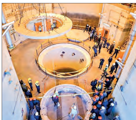
A handout picture provided by Iran's Atomic Energy Organization in December 2019 shows the nuclear water reactor of Arak, south of capital Tehran. PHOTO: ATOMIC ENERGY ORGANIZATION OF IRAN/AFP/FILE
