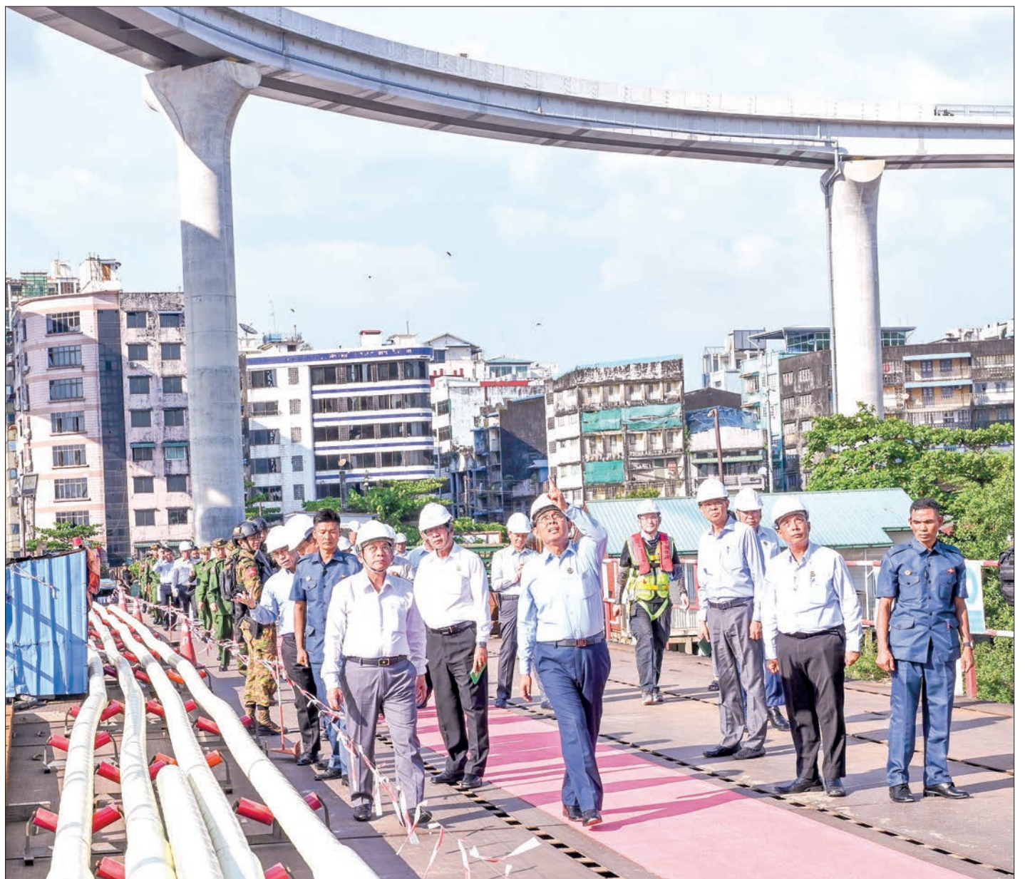
State Administration Council Chairman Prime Minister Senior General Min Aung Hlaing views round the construction project site of the Myanmar-Korea Friendship (Dala) Bridge yesterday.
