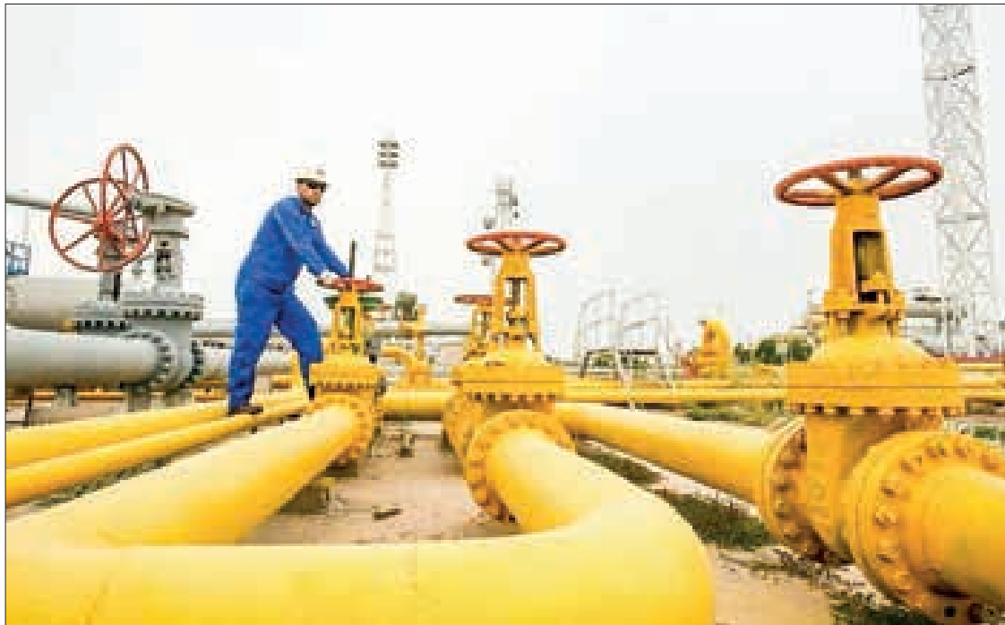
Iran's oil infrastructure is a crucial component of its economy, comprising a network of production, refining, and export facilities. PHOTO: AFP/FILE
