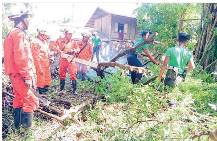
Post-flood cleanup measures are underway.
