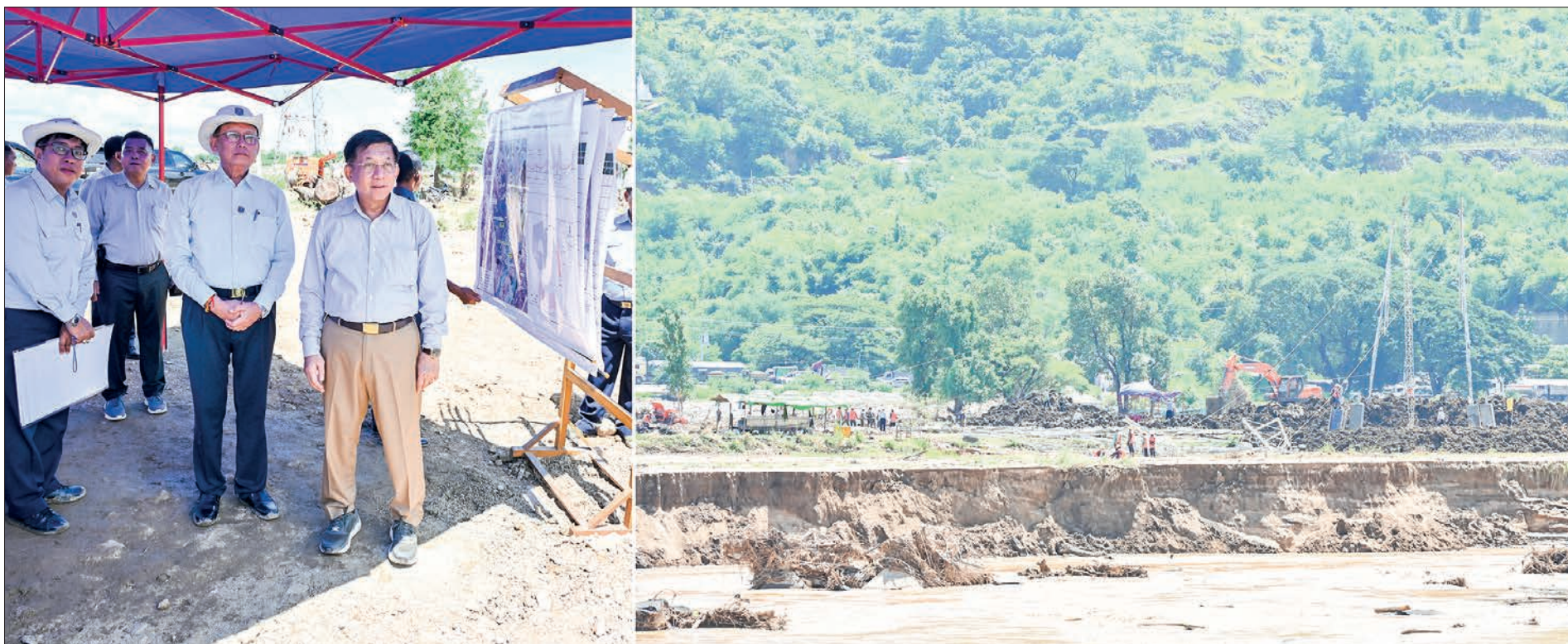
Chairman of the State Administration Council Prime Minister Senior General Min Aung Hlaing inspects the repair work of five fallen towers along the 230 kV Thazi-Shwemyo national grid near the Kintha junction in Nay Pyi Taw Council Area yesterday.
