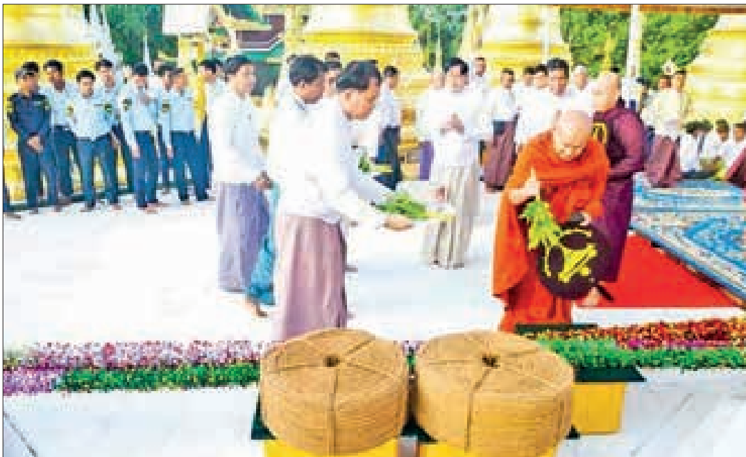
Preparations are underway to build a scaffolding structure. PHOTO: SHWEDAGON PAGODA BOARD OF TRUSTEES
