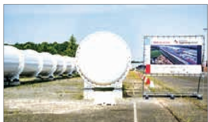
The view depicts the end of a Y-shaped tunnel measuring 420 metres (1,377 feet) at the European Hyperloop Centre in Veendam, highlighting advancements in Hyperloop technology. PHOTO: AFP
