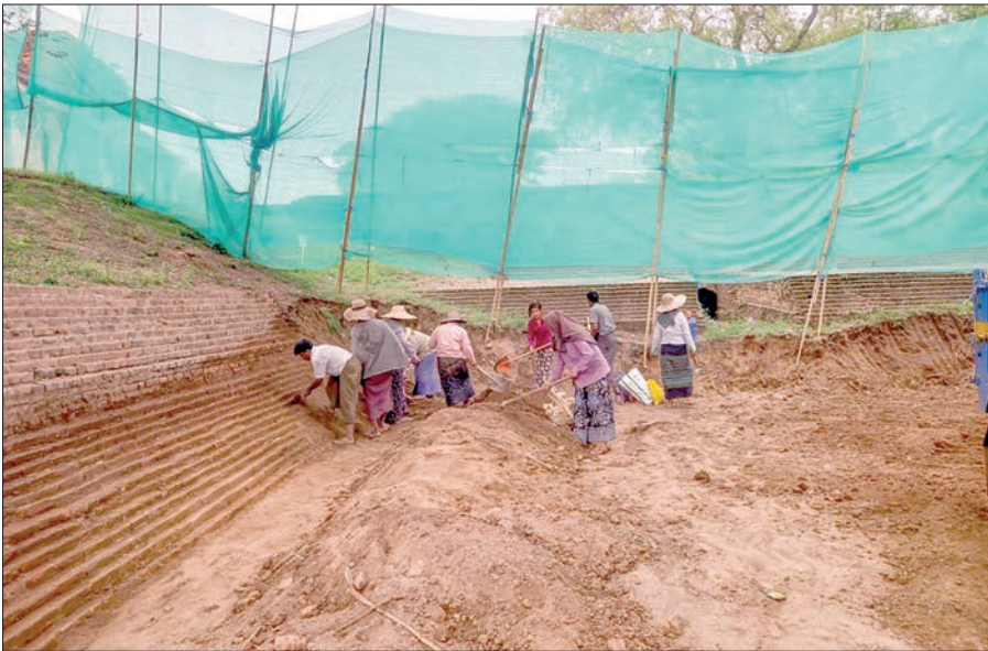
Excavation and maintenance works are underway in the eastern part of the moat of King Pyinpya's Palace.
