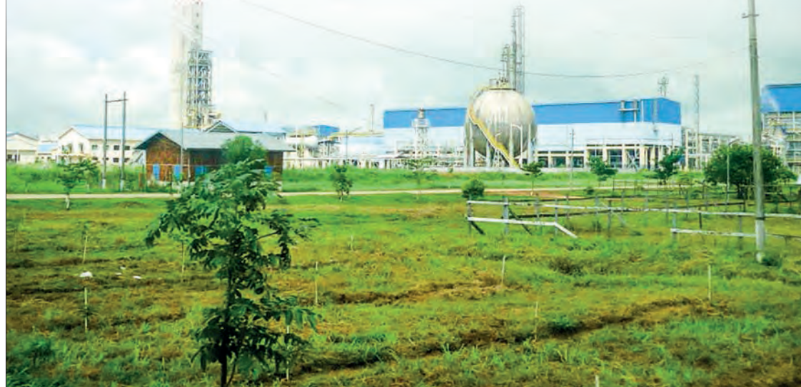
A general view of No 4 Fertilizer Plant in Myaungtaga, Hmawby Township, Yangon Region.
